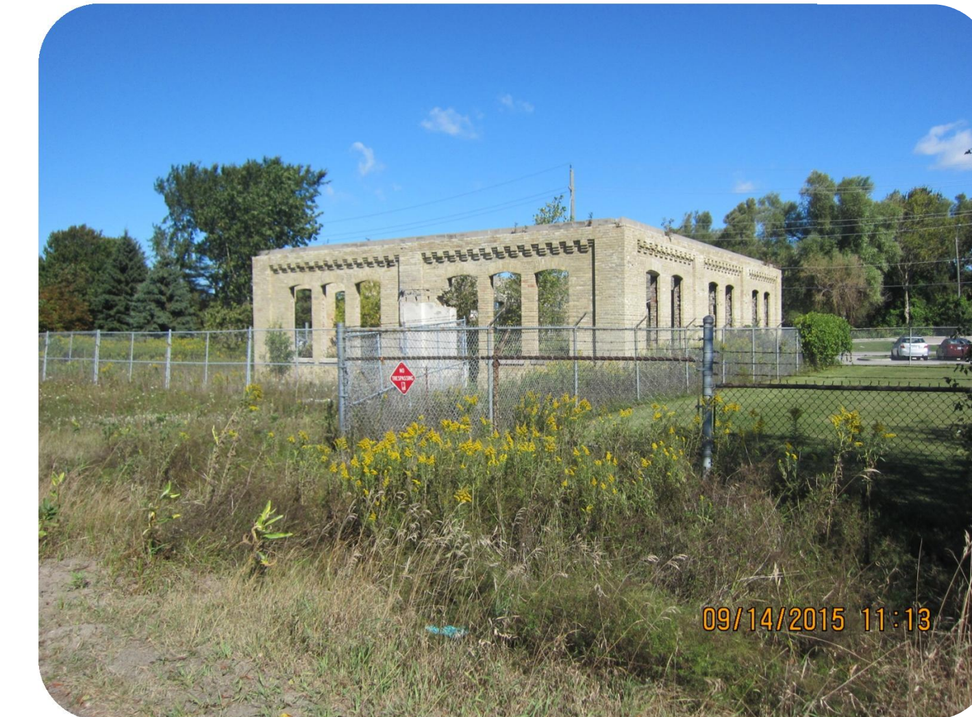
Old Stone Pump House
