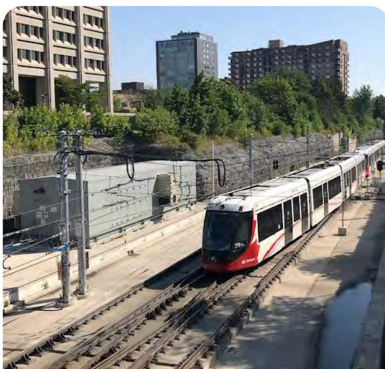
Power Substation Ottawa LRT
