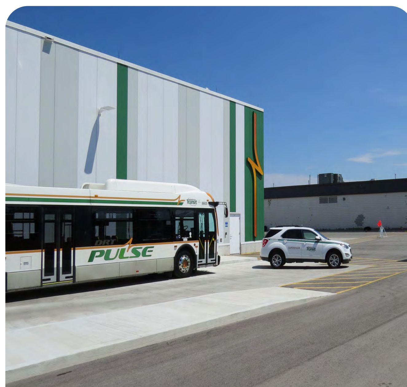
Existing DRT Maintenance Facility
