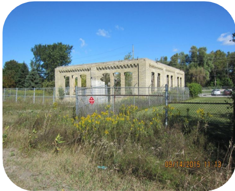
Old Stone Pump House
