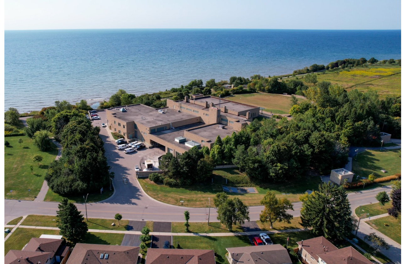
Figure 1: Ajax Water Supply Plant, 75 Lake Driveway East, looking southwest
