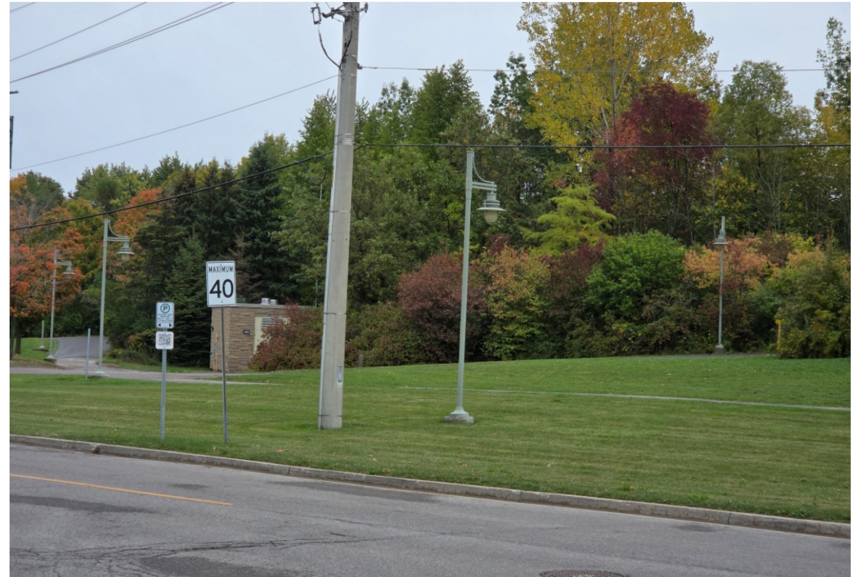
Figure 15: Lakeshore Sanitary Sewage Pump Station, looking southwest
